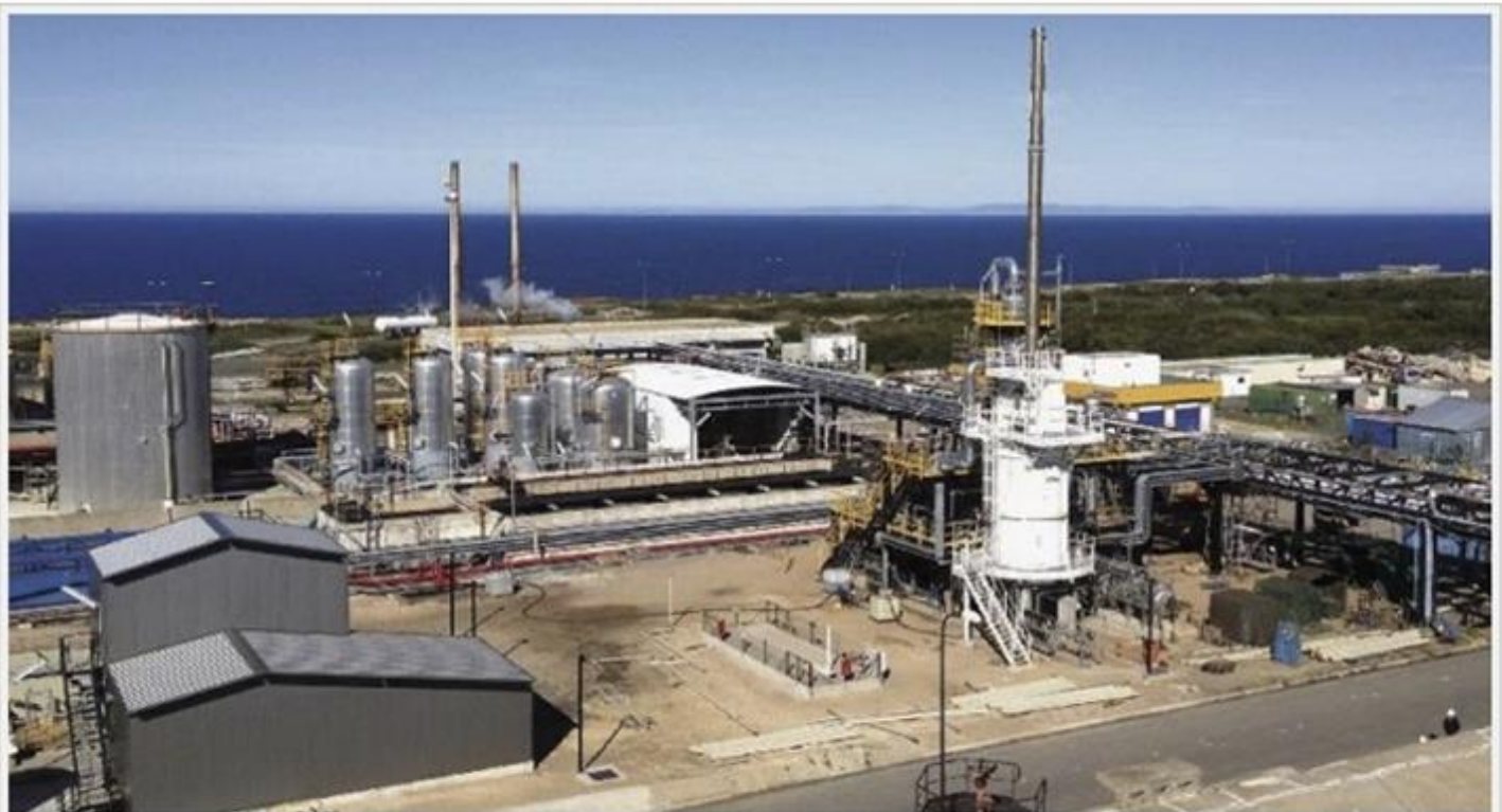
Ecoslops' refinery in the Port of Sines, Portugal. Photo: Ecoslops
